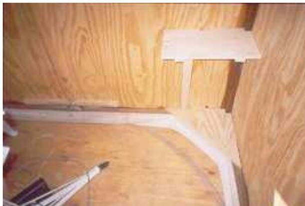
This last picture shows one of these triangular corner sections, a little work table mounted in the corner, one of the pier legs, a castor mounted in the middle of one of the sides, and some skirting at the bottom made from canvas, that drags across the floor when the dome is rotated, to prevent dust blowing in from outside. The interior sides and roof were left untreated. The floor, however, was painted top and bottom with polyester resin for waterproofing.
