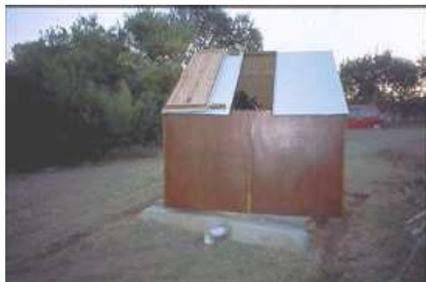
The open slit is visible here. The slit is wide enough so that the scope can track for about an hour, which means that there is no need for automatic rotation of the dome. Although I sometimes have to nudge the dome a little from outside. The pipe is obviously used for power and signal cabling between the observatory and the computer in the shed.
