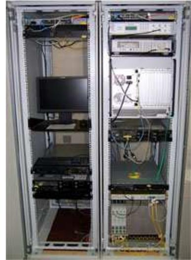
The RF signal connects to the back end receiver via the unit in the bottom right. These two racks contain the digital receiver, the PC running the analysis software and all of the telescope control PCs.
