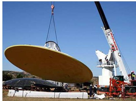
The composite dish being lifted from the mould, to be fitted to the antenna positioner.
